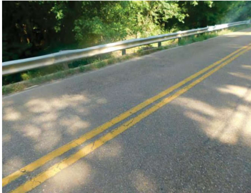
VIEW ACROSS TOP OF DECK
