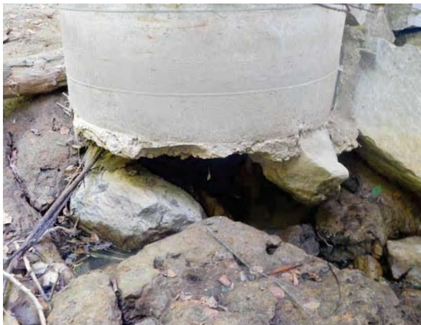
PILE A BENT 1 WASHING UNDER CASING
