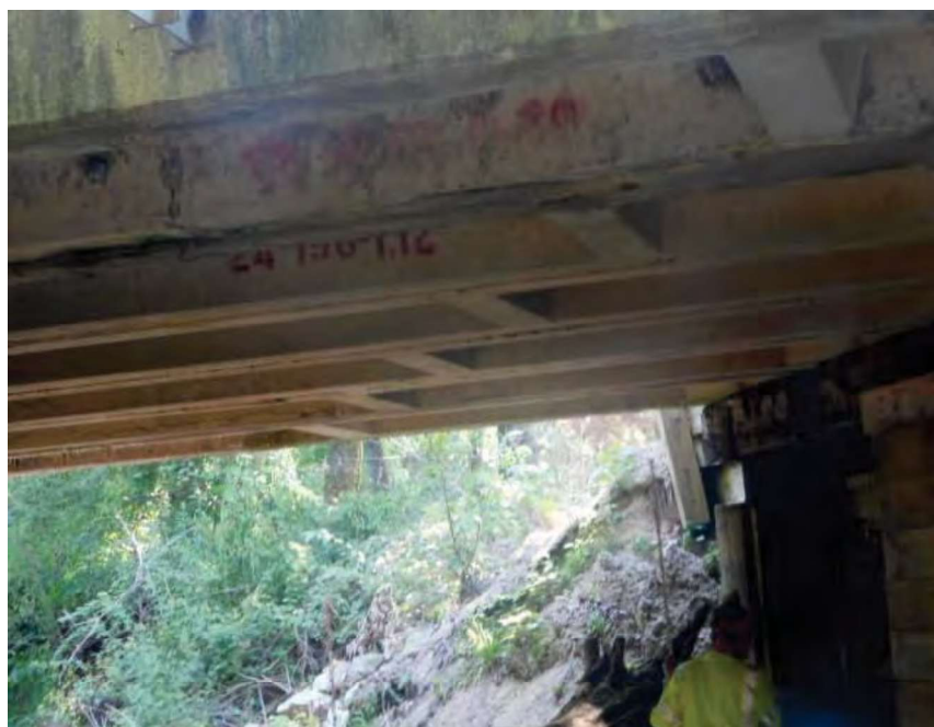
BOTTOM DECK SPAN 1
