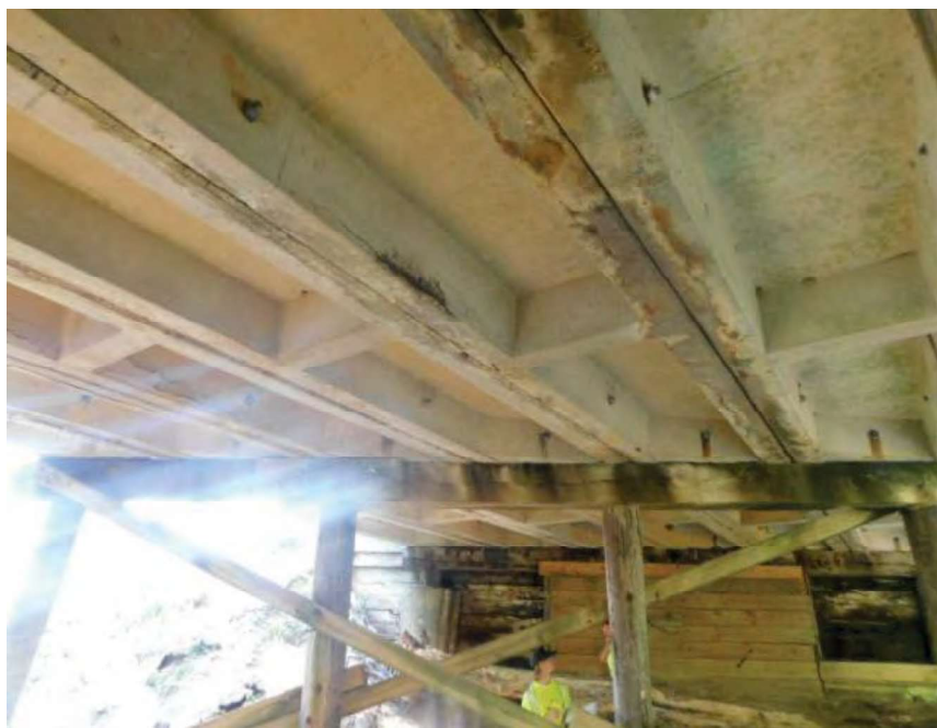
BOTTOM DECK SPAN 2
