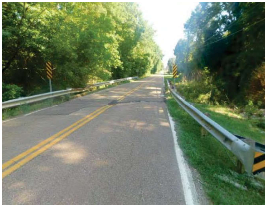
LOOKING AHEAD ON ROUTE
