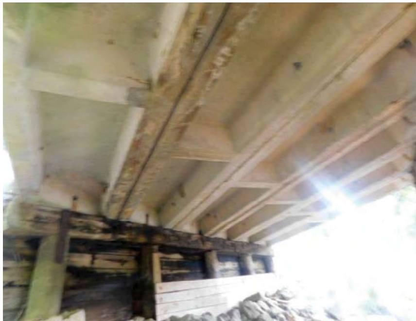
BOTTOM DECK SPAN 3
